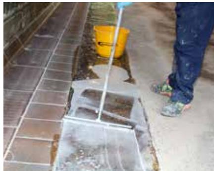
**Tip:** Individual deeper holes (max 5cm) can be filled selectively: simply mix 1 part primer with 2 parts of quartz sand (<math>0.9\text{ mm}</math>) and pour into holes or fill.
