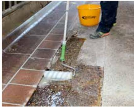
The coating basically starts with the thin application of the **primer**. It ensures secure adhesion.
