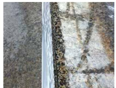
Masking the area to be coated with stone tape, preferably before the last coating. Remove the tape about 30 minutes after coating.
