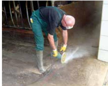
Cut a boundary groove of approx. 3 mm depth with the diamond disc as the final edge.
