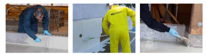
After priming, apply **Top-F** to the concrete back walls of feed tables and silo walls with a roller.
