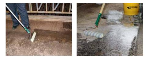
The underground surface must be primed with **PowerGrip** before further coating to create an optimum bonding bridge. To do this, mix the 2 components of **PowerGrip** homogeneously, decant in fresh bucket, mix again and then apply with a roller. Let the primer dry.
