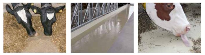
Finished surfaces are suitable for use with feed after 2 days, full chemical and mechanical resistance is achieved after 7 days.
