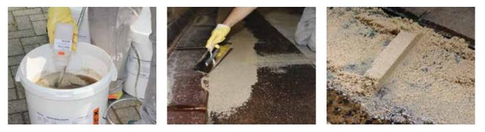
Very severely damaged floors must also be prefilled with **easyFill** before coating with Basic. This creates a flat surface and saves material and grinding work. Mix the mineral mass with resin and hardener in a bucket. Apply the compound with a spatula and a smoothing trowel. For good compaction, tap firmly.
