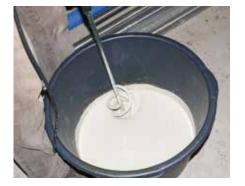
Mix the 2 components of **Basic** homogeneously and then **transfer** into another bucket and **mix again**.
