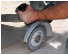
In order to obtain a perfect finish to the foot antenna, use the diamond wheel to cut a limiting groove of 3-5 mm depth along the edges of the feeding table.
